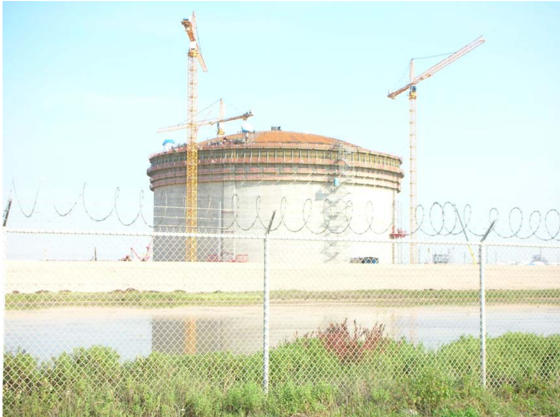
Fig. 2: Completed Liquid Nitrogen Gas Tank
